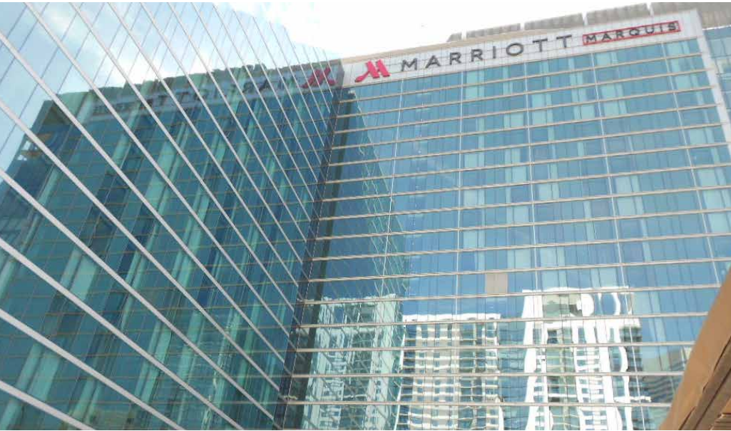
The Marriot Marquis Houston, TX | 1,000 Rooms
