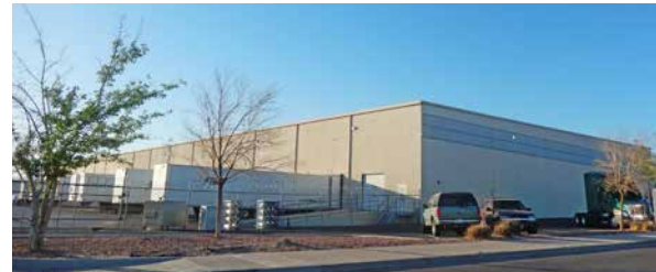
Escobar Distribution Center Houston, TX
