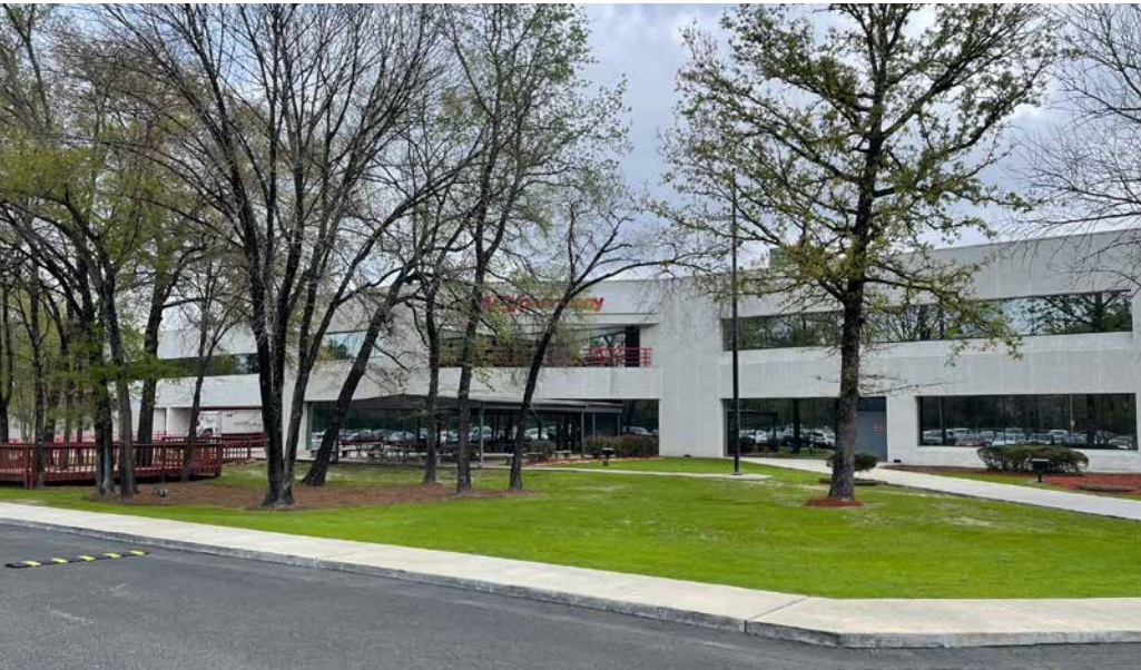
CVS Distribution Center Conroe, TX
